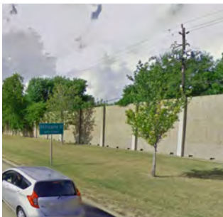
Beltway 8 Frontage Road North of Phillipine
